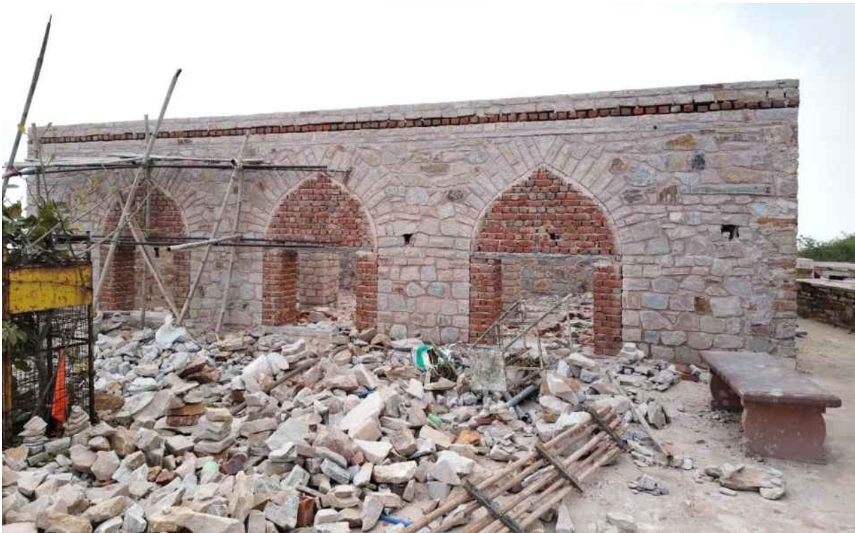
During Construction of a sculpture shed at Harshnath (work in progress)
